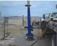
**Horizontal**: Attach **BORELINE** to vehicle and lower into well.
